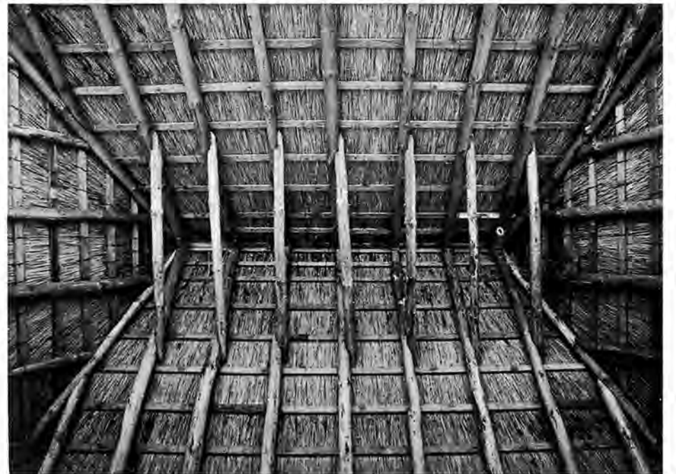
POLE ROOF FRAMES AT NETHERLANDS OPEN AIR MUSEUM, ARNHEM, HOLLAND
