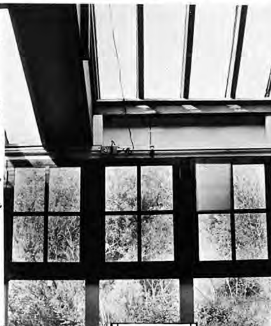
USED LEADED GLASS WINDOW REHUNG ON USED WOOD FRAME.
