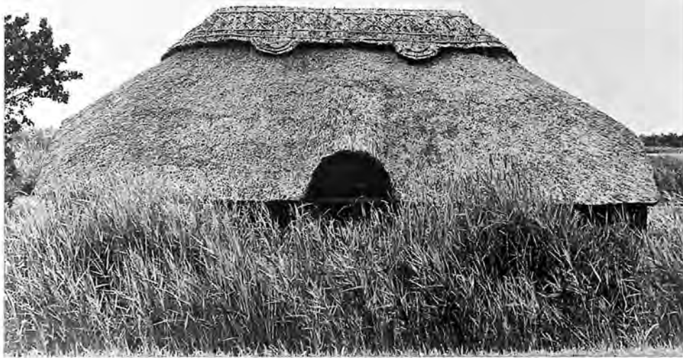
NORFOLK REED ROOF ON BOAT SHED, NORFOLK, ENG.
