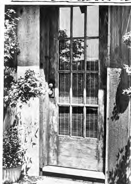
USED FRENCH DOOR REHUNG ON NEW USED WOOD FRAME.
