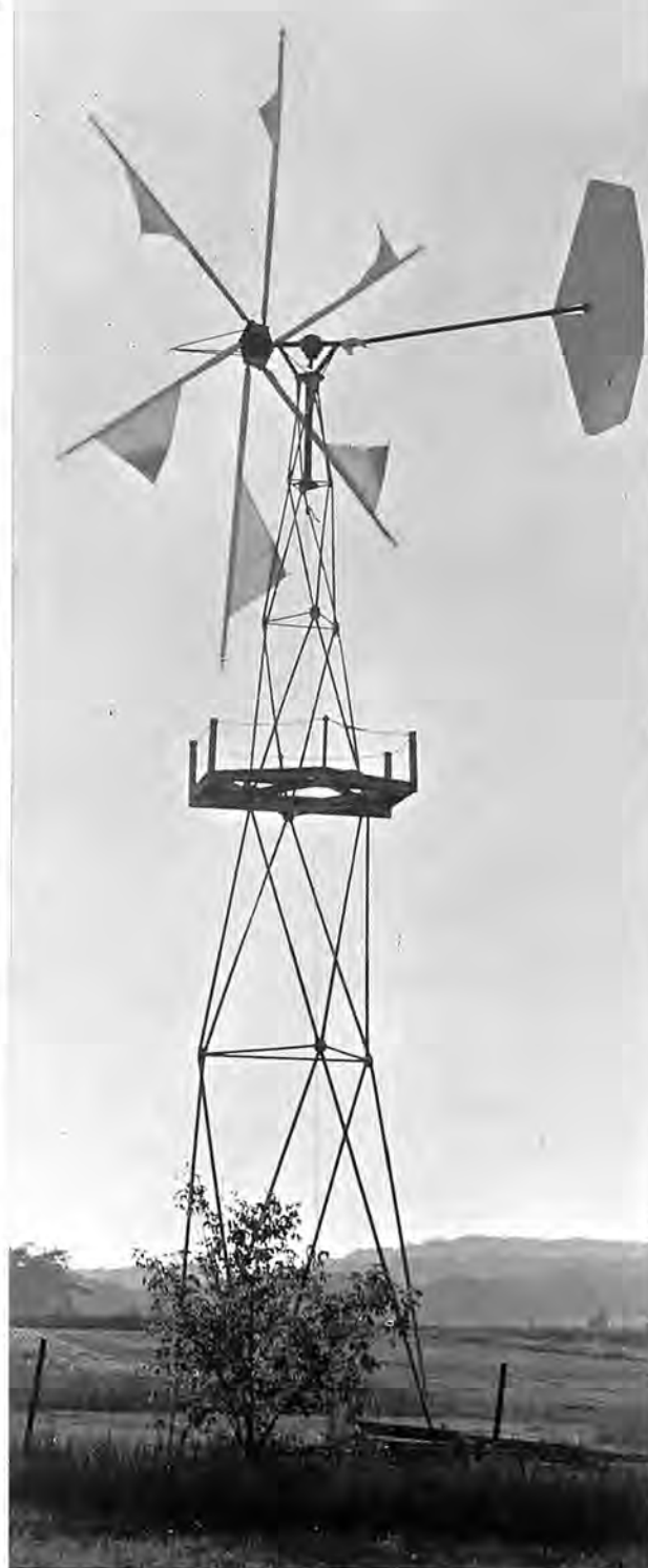
Windworks sail windmill, 1974. Since the photo, driveshaft to base has been added to drive buzz saw and electric generator.
