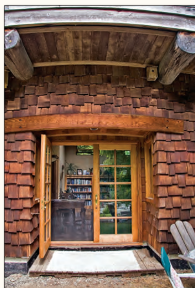
Exterior finish in traditional cedar shakes
